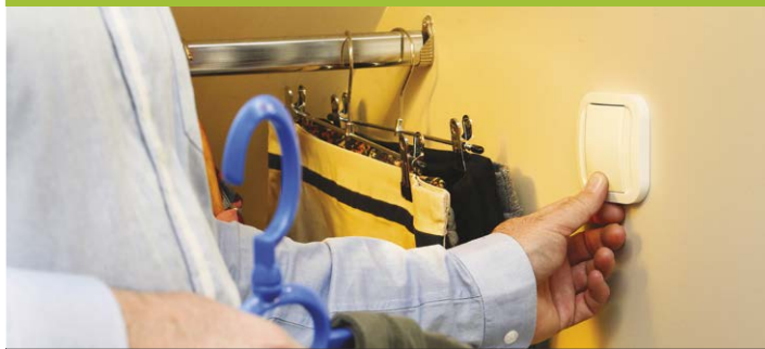
Creation of a new back-and-forth with a wireless and battery-less wall switch
